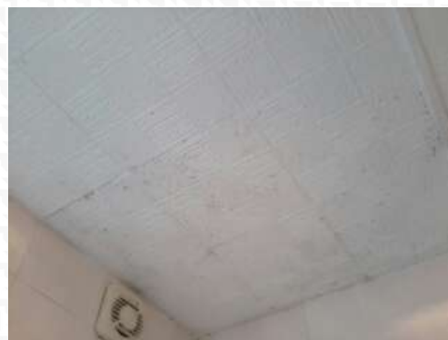
Mould spot stains to ceiling
